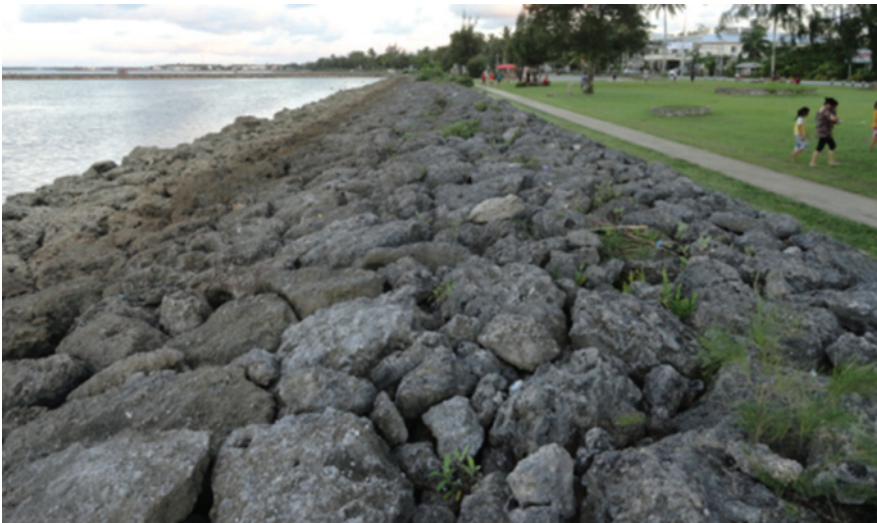
Figure 36: Rock revetment, Nuku'alofa
