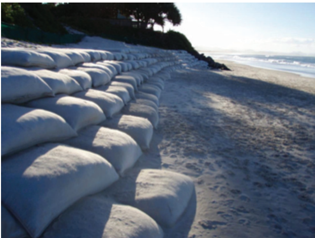
Figure 38: Sand-filled geotextile container revetment at Byron Bay, New South Wales, Australia
