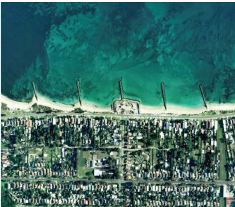
Figure 41: Groynes at Botany Bay, New South Wales, Australia
