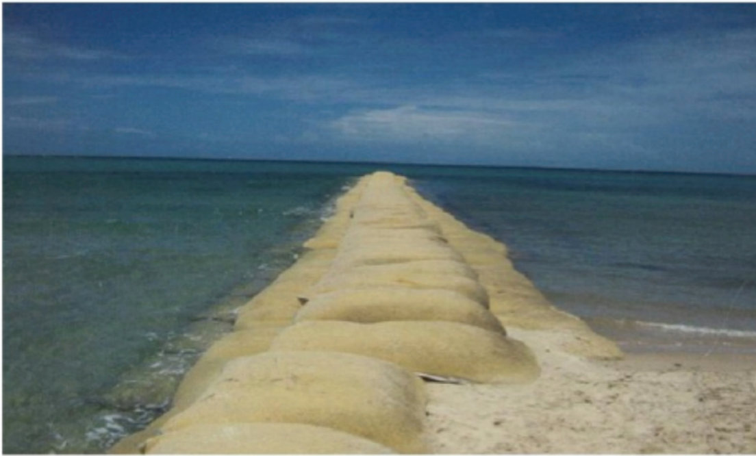
Figure 42: Groyne made of geotextile bags
